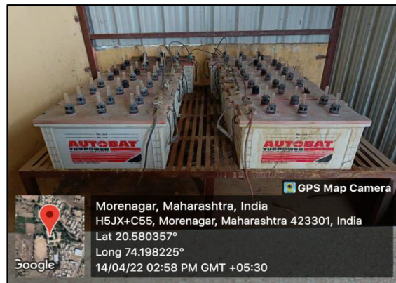
Photo: Batteries Connected for off grid System
