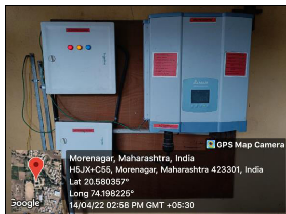
Photo : DC Distributor Box and Complete Installed off grid unit.
